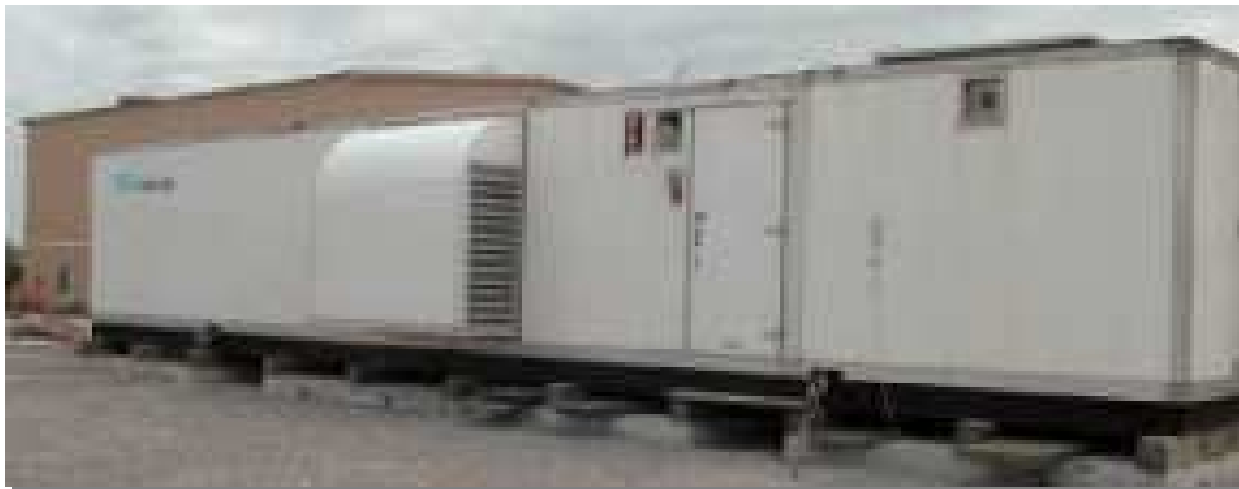
Figura 6.47. Micro-SMES (6 MJ, 750 kVA) (Intermagnetics General Corporation).
